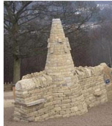
Within the exhibit, a circular pinfold half buried in the hillside displays the skills involved in building in a tight curve, and a set of demonstration walls show the various stages in building in dry stone. Different styles of topstone reflect the styles found in urban and rural landscapes, including half rounded topstones and "cocks and hens".
