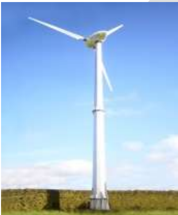
10kW wind turbine (15m mast) located near Bradshaw
