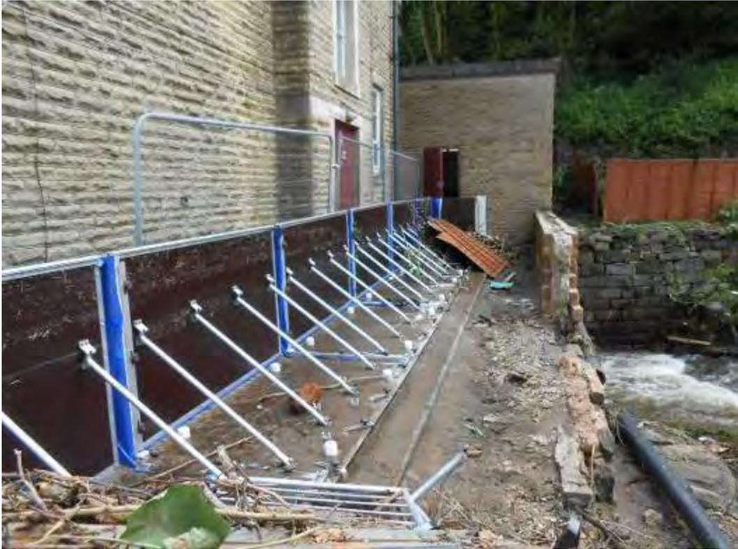
Figure 6 – Damaged caused by flood waters on the new unfinished flood wall being constructed. During the flood event a section of the temporary works collapsed, reducing the capacity of the channel. The constriction at the culvert caused an increase in the level of flood waters upstream of the culvert. Approximately 50 metres upstream is a small, privately owned, masonry vehicle access bridge which suffered structural damage resulting in the collapse of the bridge parapet and masonry facing.
