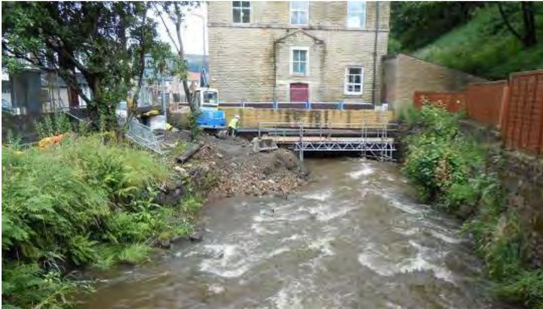
Figure 5 – View looking downstream at the temporary construction works on the culvert on the Walsden Water.
