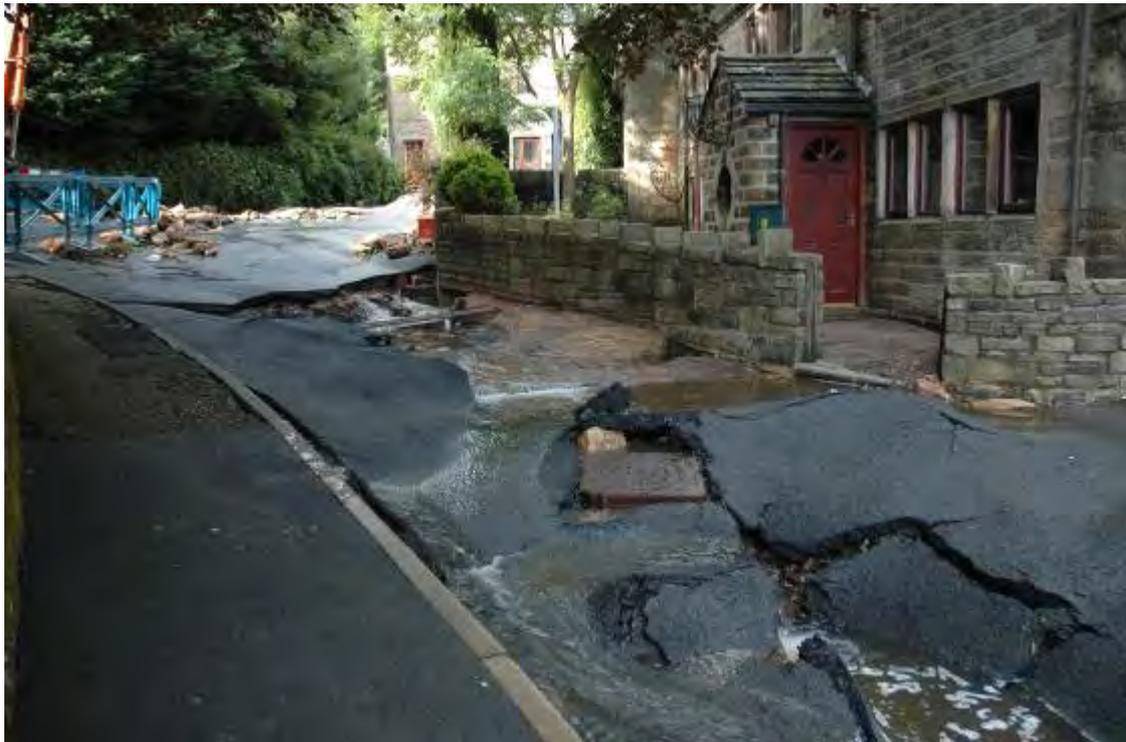
Figure 3 – Kershaw and Clough Road, road surface severely damaged as a result of the excess surface water on Clough Road.
