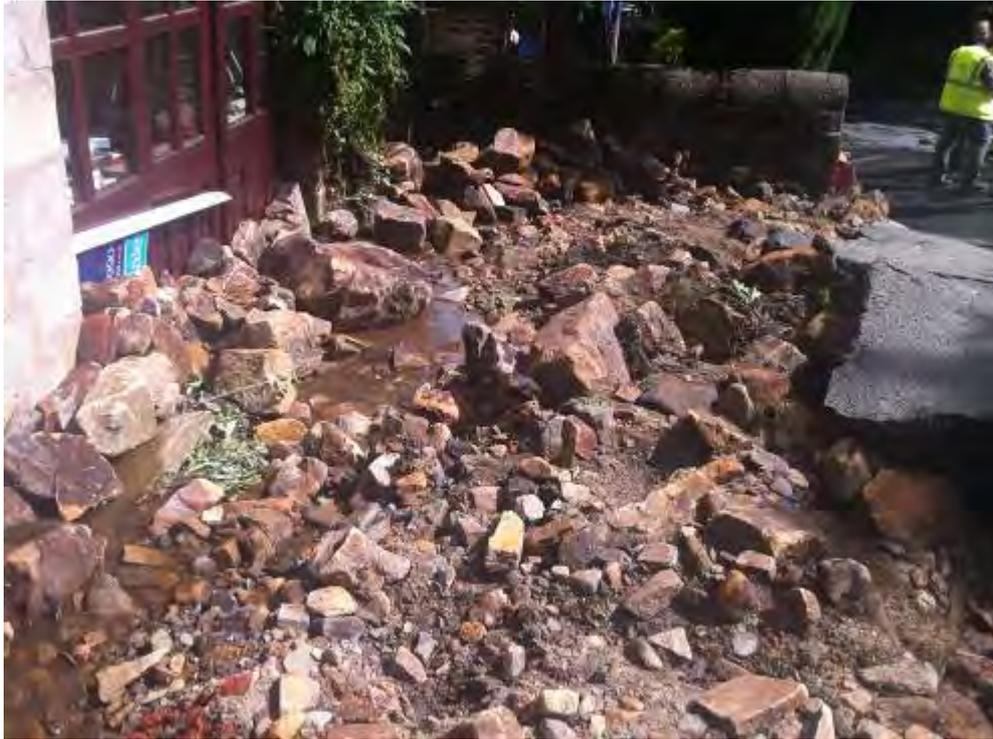
Figure 2 – Debris from the collapsed culverts onto adjacent property
