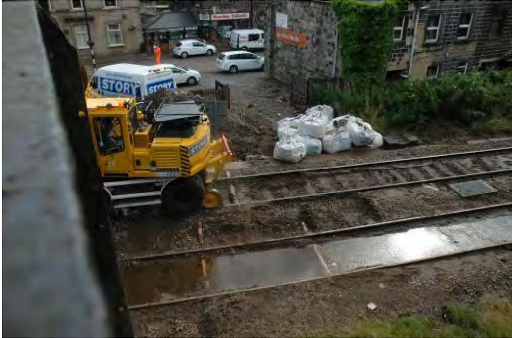
Figure 9 – Network Rail repair teams removing large volumes of debris and reinforcing rail track immediately after the flood event.
