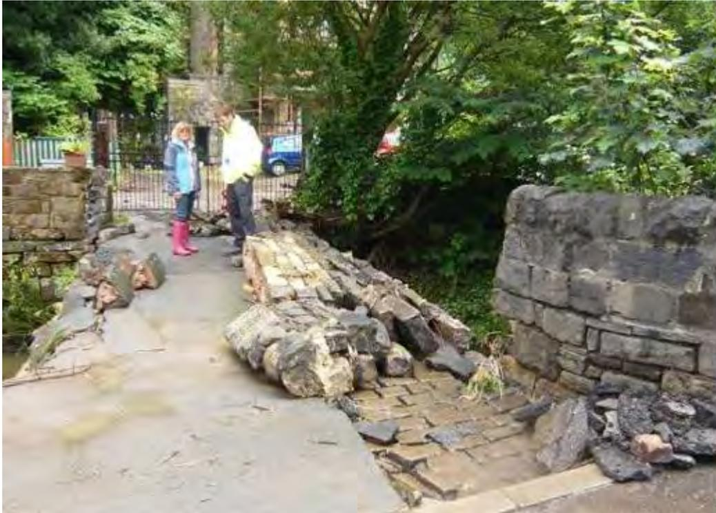
Figure 7 – Damage to the bridge and parapet walls after the flood event on an access bridge on the Walsden Water.
