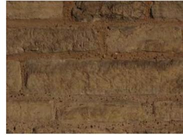
Cement mortar must not be used as water cannot pass through the impermeable joints and becomes trapped in the stonework. As the water freezes in winter it expands and causes the surface of the stone to fall away. Over time this causes significant damage.
