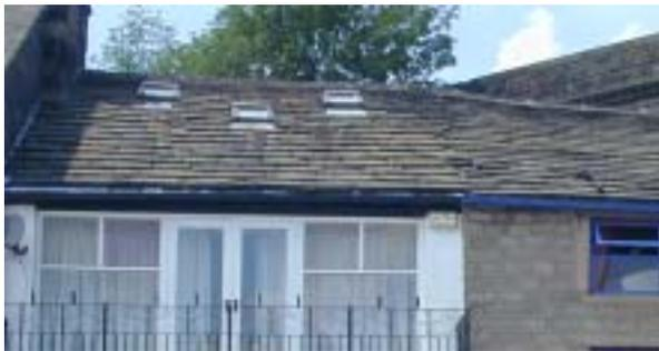
Local stone slates - sometimes laid in slightly diminishing courses with smaller slates to the top, gradually increasing in size further down the roof
