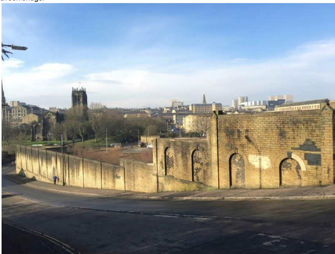
Figure NTS7: View towards Halifax Minster from the Cripplegate/ Bank Bottom/ Berry Lane (E07/08/09B) intervention. The Cripplegate site will be used as a temporary construction compound.
