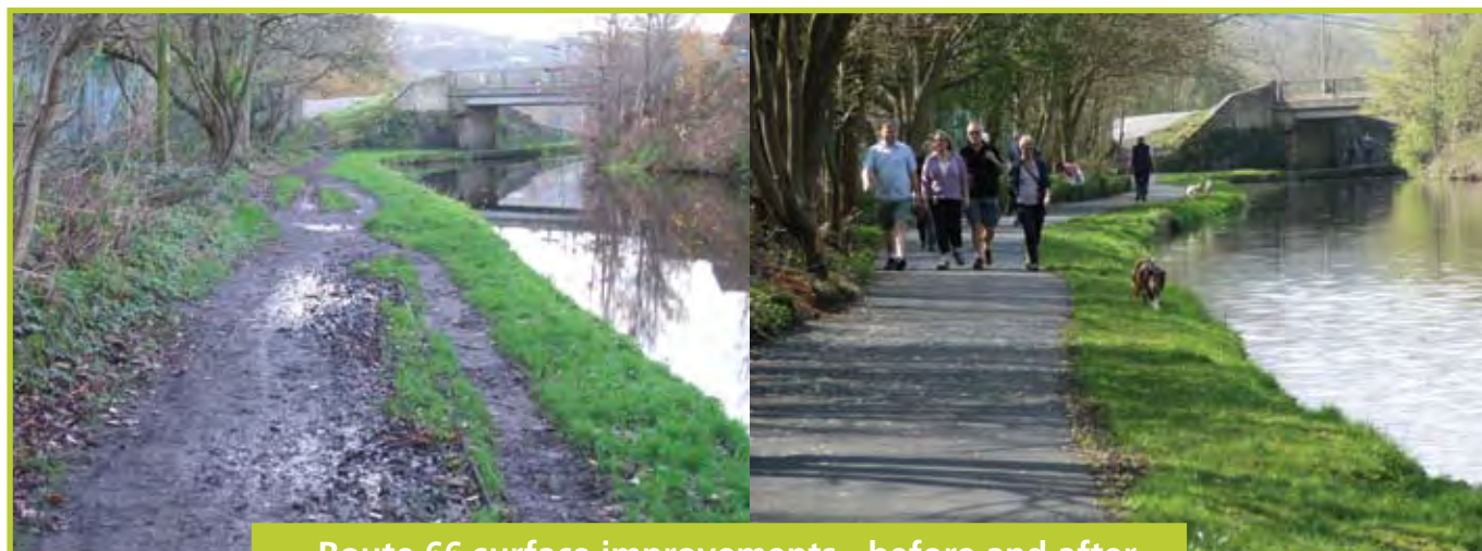
Route 66 surface improvements - before and after
