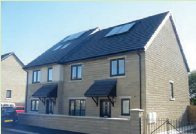
New houses at Upper Parkinson Lane, Halifax
