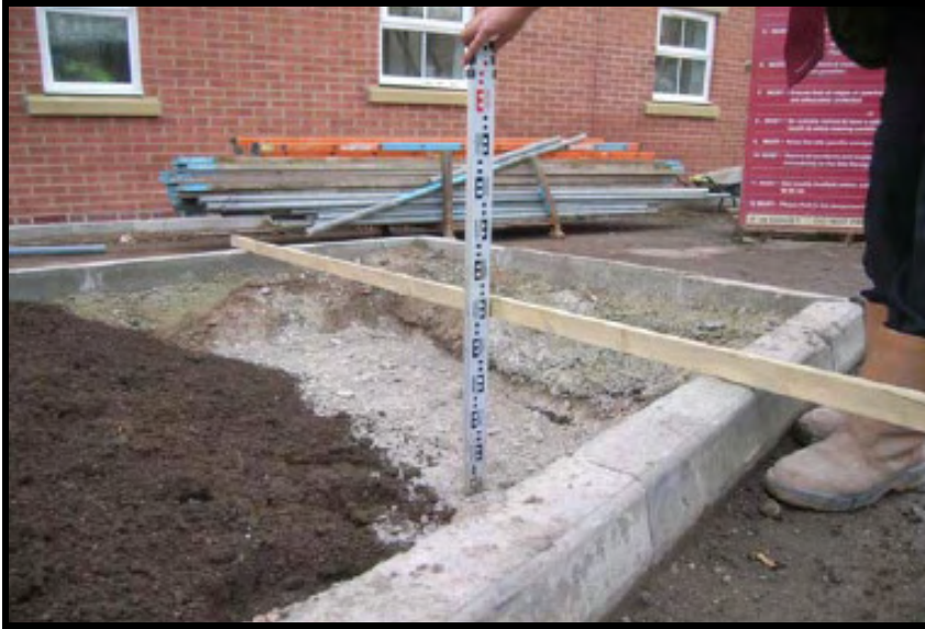
Photograph 1 : Depth check of inert cover within area of public open space. Physical break layer and topsoil visible.
