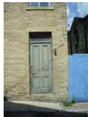
Rough finished irregular coursed masonry (Sowerby Bridge town centre)
