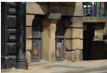
Rusticated ashlar masonry (Sowerby Bridge)
