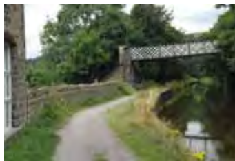
Pedestrian footbridge over the canal.
