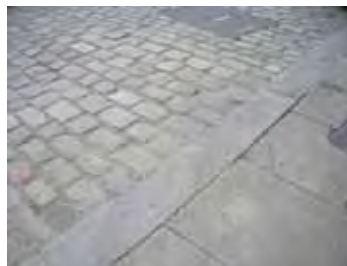
Contemporary granite setts with yorkstone paving.
