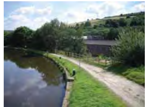
Existing building on the Holmes Road site with the Rochdale canal in foreground.
