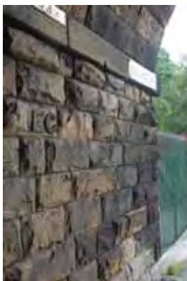
Riven faced stone with regular coursing (Holmes Road railway arch)
