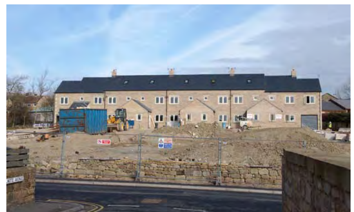
View of construction of Clovecroft
