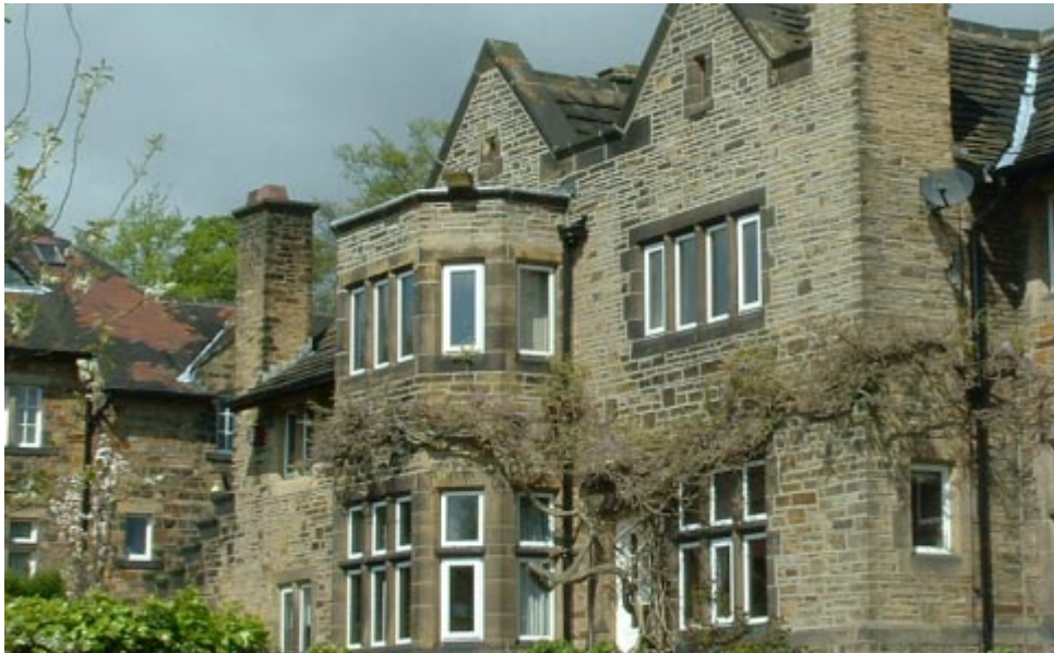
The Croft, designed by the architectural practice of Walsh and Nicholas
