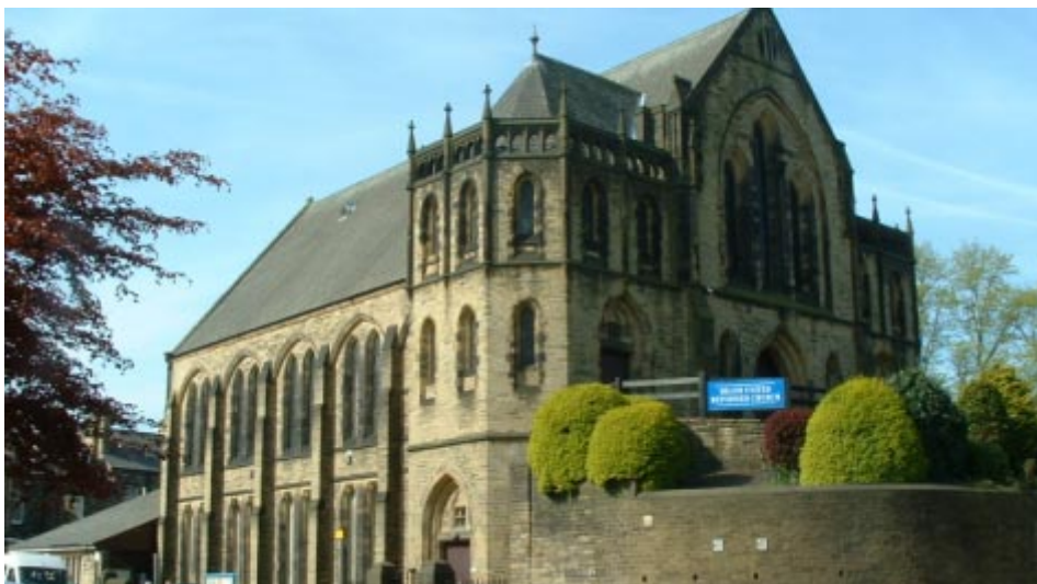
View of Heath United Reformed Church from Free School Lane
