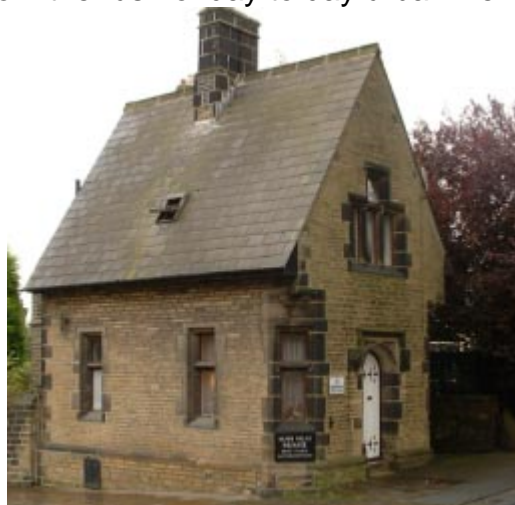
Entrance Lodge, Heath Villas
