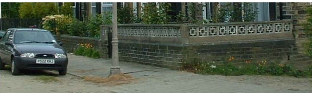
Boundary walls altered by adding concrete blocks
