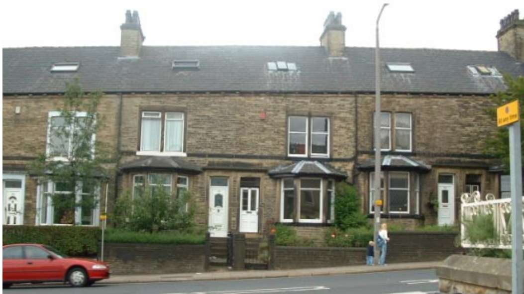
Huddersfield Road looking from Stafford Square
