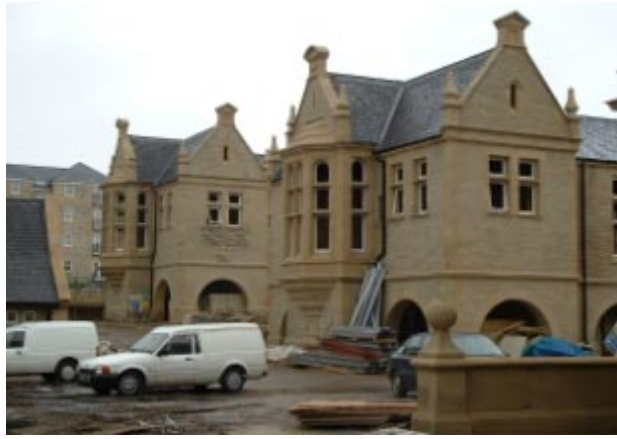
Conversion of the former Royal Halifax Infirmary to flats in 2004
