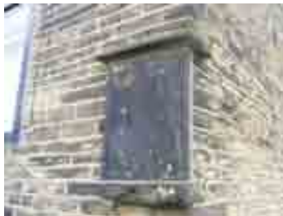
Examples of weathered local coursed sandstone
