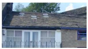
Local stone slates - sometimes laid in slightly diminishing courses with smaller slates to the top, gradually increasing in size further down the roof
